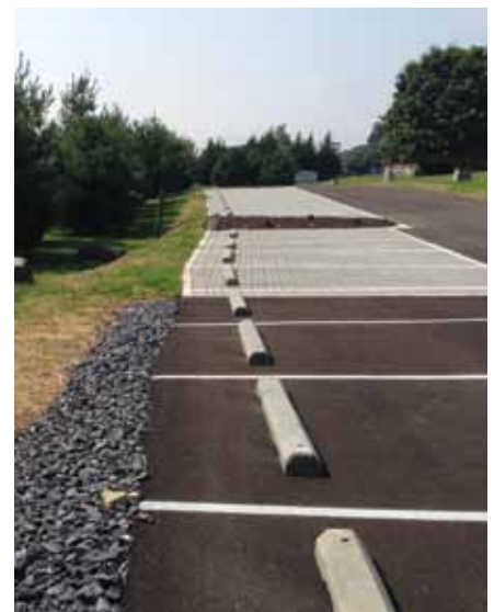
Stormwater is managed through the use of permeable pavers at this redevelopment project in Washington County.
