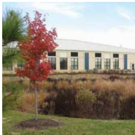
A bioretention stormwater management pond protects water quality in Talbot County.
