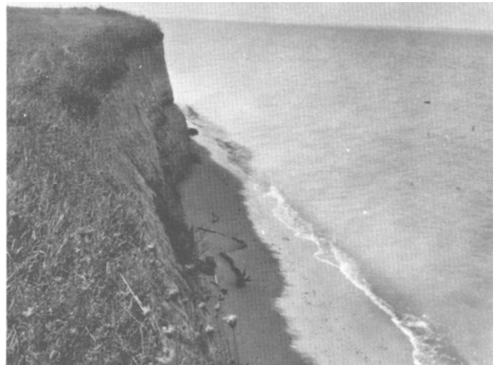
The problem of shore erosion and its control received considerable attention during Mr. Denny's Administration.
